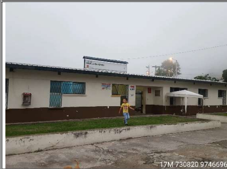
FOTO No. 92. HOSPITAL MIGUEL LEON BERMEO, CHUNCHI.
